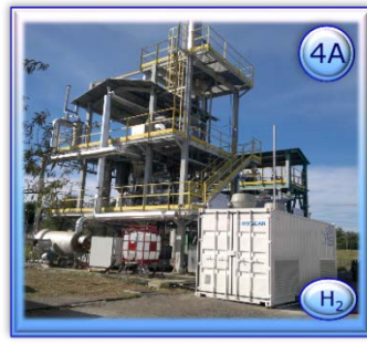
4A) Internally Circulating Fluidised Bed Steam/O 2 Gasification Plant (1 MW th ) with integrated Catalytic Ceramic Candles system for In-Situ gas filtration and conditioning. 4B) Scheme of reactor (2) .
