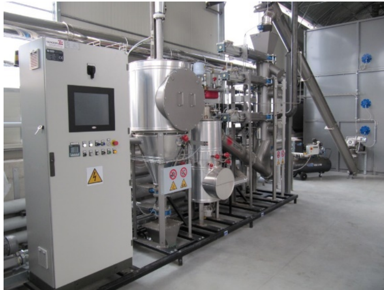
Figure 30. 49 kW electrical and 110 kW thermal cogeneration system for a greenhouse.
