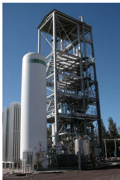
Figure 22. Demo-scale fixed-bed gasification unit (5 MW th )
