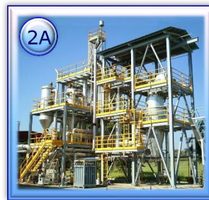
2A) Dual Fluidised Bed Steam Gasification Plant (500 kW th ) with Hot Gas Cleaning via an Adsorbing Reactor and a Filtration Unit: Cyclone plus Ceramic Filter. 2B) Scheme of reactor (1) .
