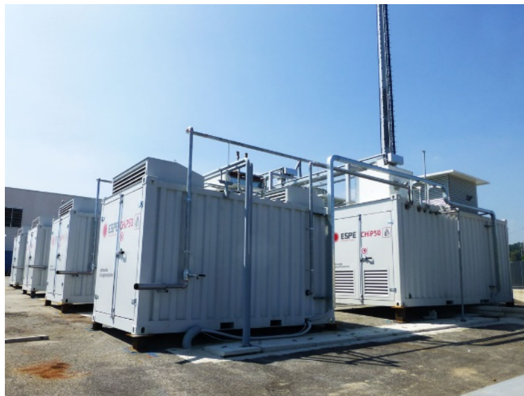
Figure 31. 196 kW electrical and 440 kW thermal cogeneration system containerized unit for heating and drying processes
