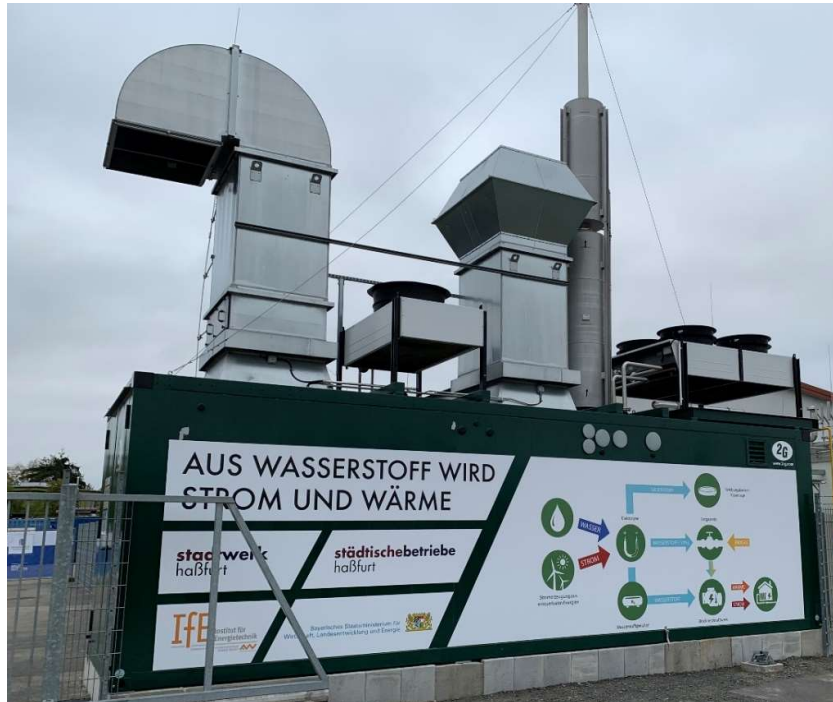
Figure 18 The hydrogen powered CHP unit in Haßfurt
