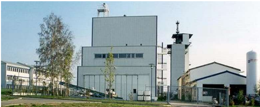
Figure 159: FlexiEntrained gasification pilot plant in Freiberg
