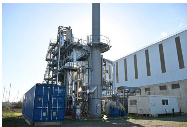
Figure 13 - Leroux&Lotz Innov'Energy platform near Nantes (picture: Leroux&Lotz)
