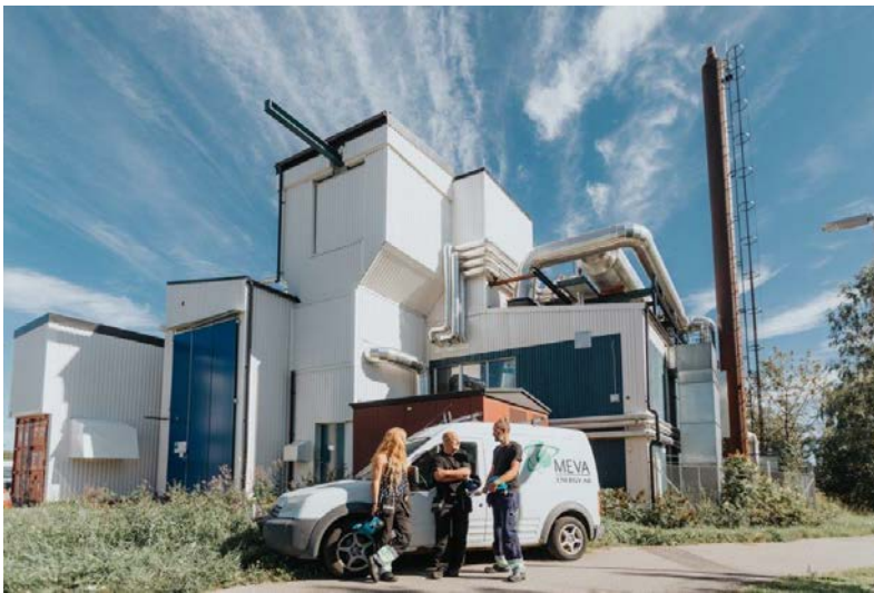
Figure 21. The Meva gasification plant in Hortlax.
