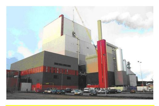
Figure 2: The Amer-9 coal-fired power station with the waste wood gasifier (front-right)
