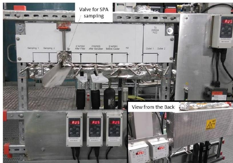
Figure 55. Central panel of new gas sampling system implemented at the GoBiGas plant [60].
