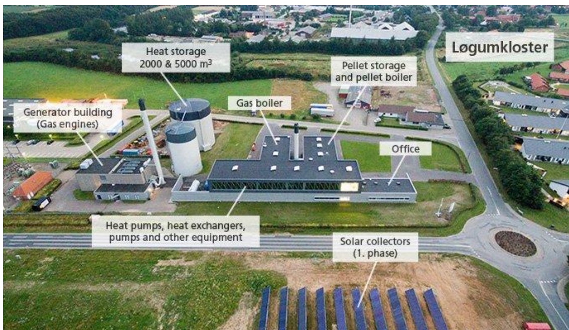
Figure 4. Hybrid district heating plant (CHP) combining wood pellets, solar thermal energy and natural gas in Løgumkloster in Denmark [18].
