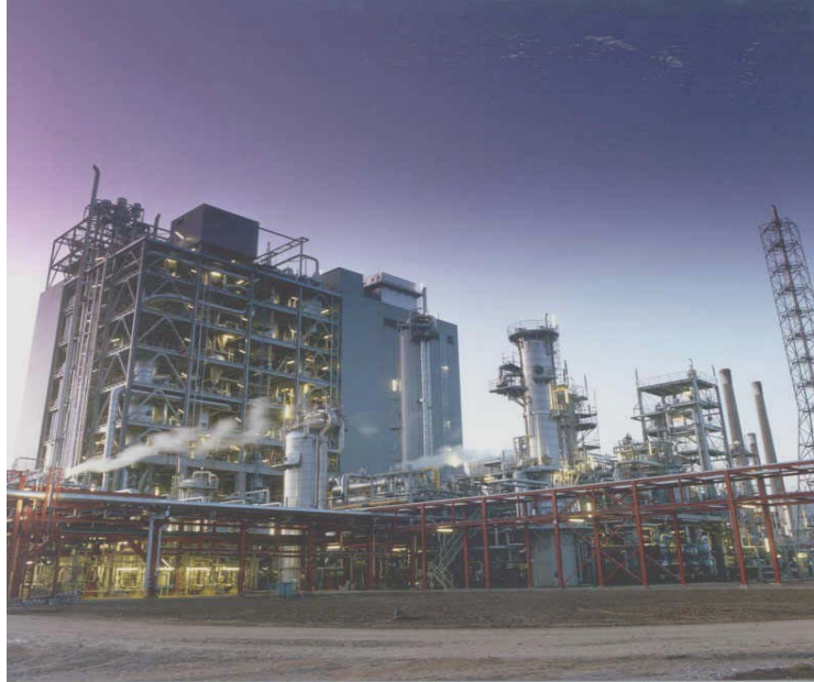
Figure 24: The Shell Entrained Coal Gasification Plant at Willem-Alexander Centrale
