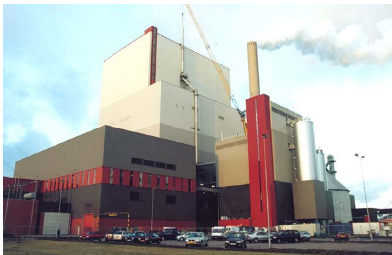
Figure 23: Essent/AMER Lurgi CFB BMG Plant (Capacity : 85 MWth biomass)
