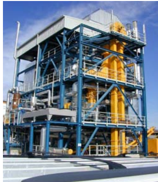
Figure 1: The TUV- FICFB Biomass Gasification Process: CHP Demonstration in Güssing (8 MWth capacity, 2.0 MWe + 4.5 MWth Heat, 50 tons/day of wood chips from forestry)
