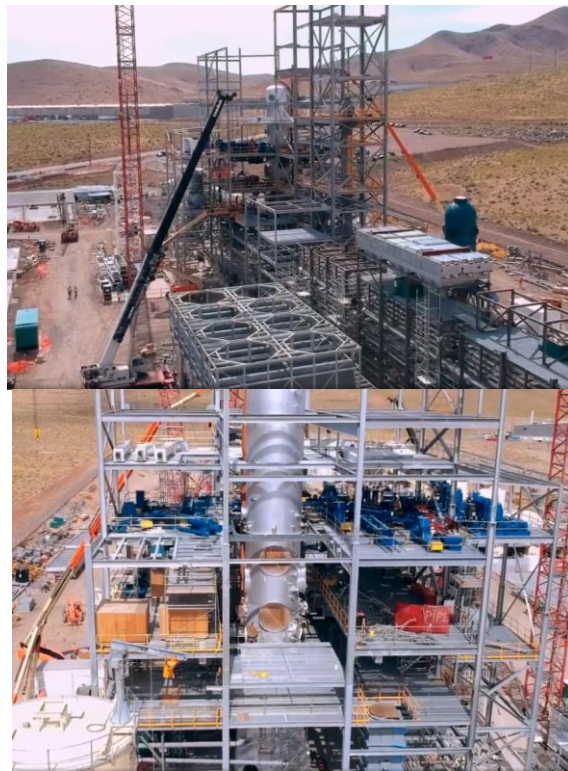
Figure 85: Construction photos of Sierra Biofuels plant. (Source: Abengoa/LinkedIn)
