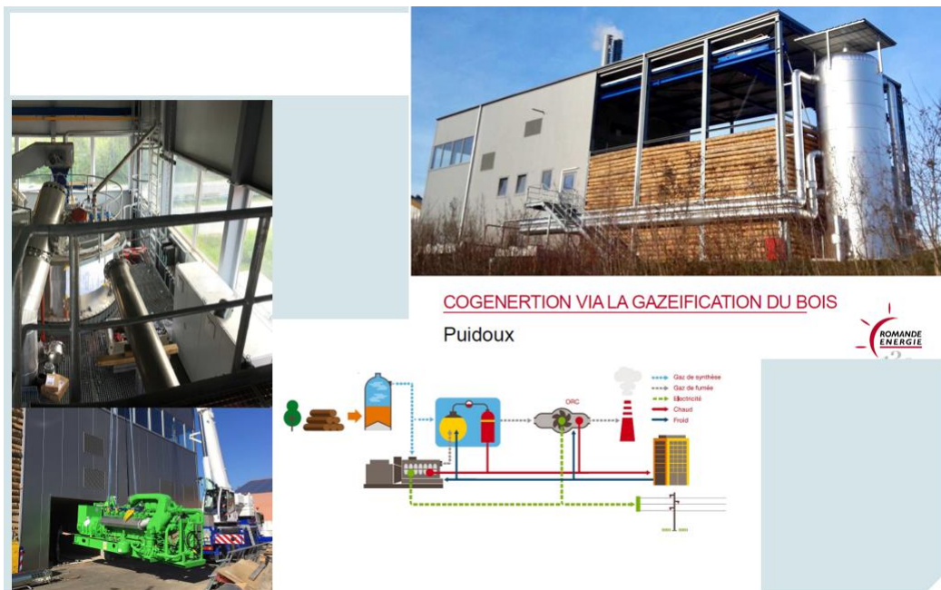
Figure 73: Regawatt unit in Puidoux
