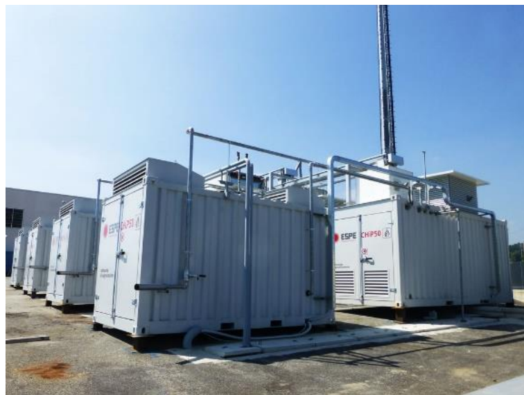
Figure 32: 49 kW electrical and 110 kW thermal cogeneration system for a greenhouse.
