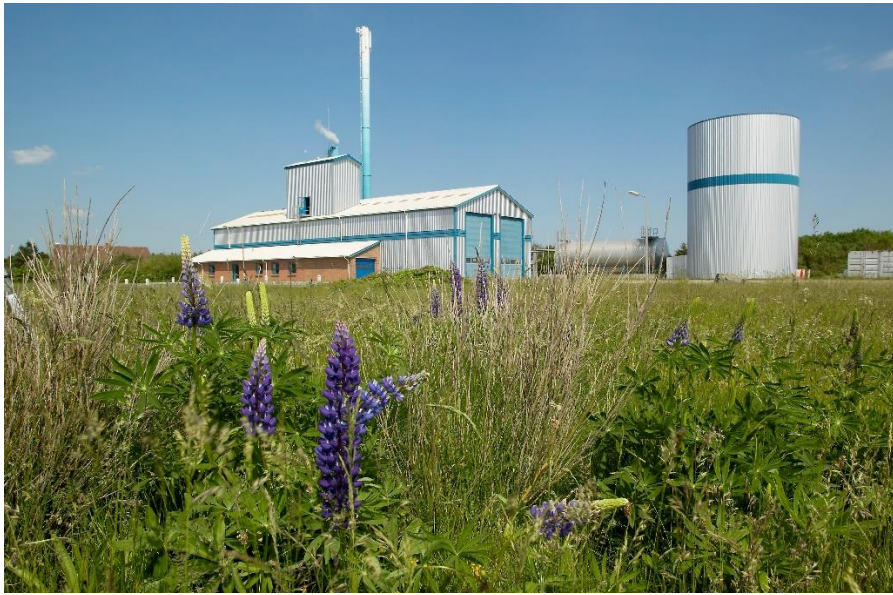
Figure 16: Photo of the gasification plant in Harboøre
