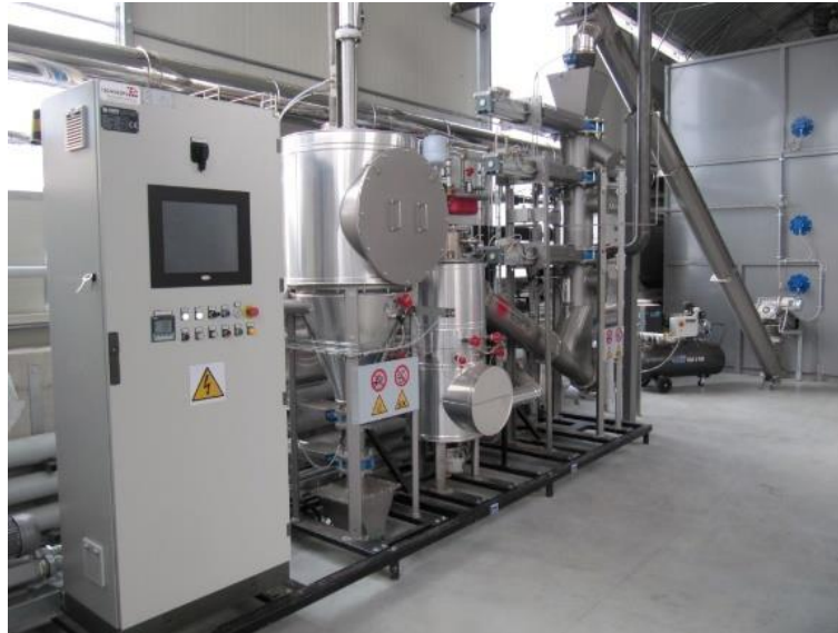
Figure 32: 49 kW electrical and 110 kW thermal cogeneration system for a greenhouse.
