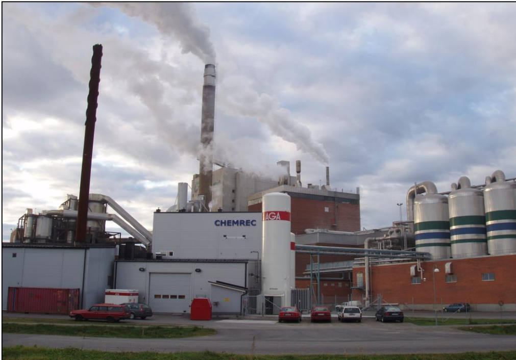
Figure 57: Pressurized development plant DP-1 at Kappa Kraftliner pulp mill, Piteå
