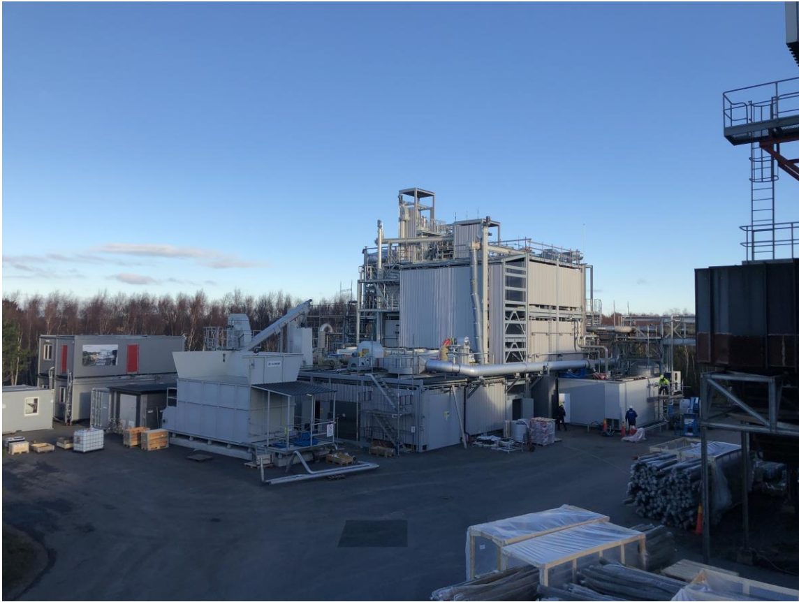
Figure 65: The ProBioStål plant at Höganäs, mid-December 2018
