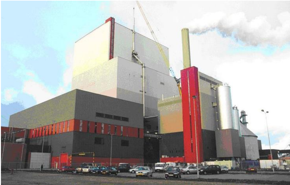
Figure 36: The Amer-9 coal-fired power station with the waste wood gasifier
