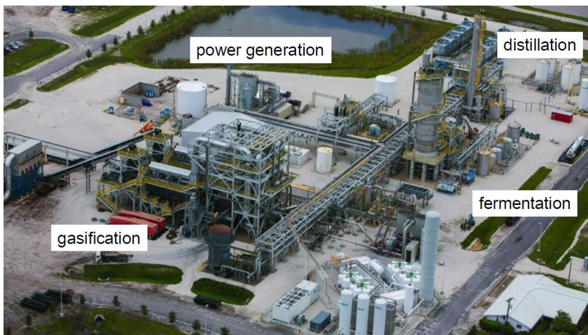
Figure 94 The INEOS Bio New Planet Indian River BioEnergy Center 587
