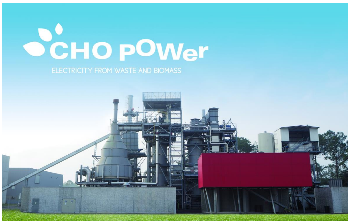
Figure 67 The CHO Power Morcenx plant 347
