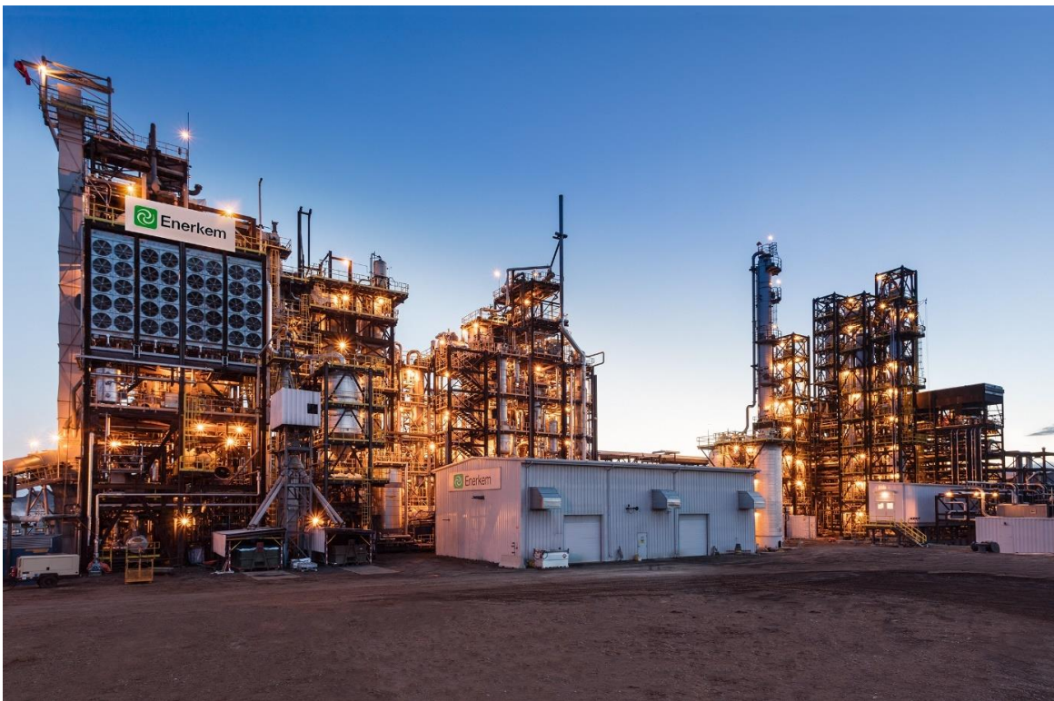
Figure 93 The Enerkem Alberta Biofuels plant 560 in Edmonton, Alberta
