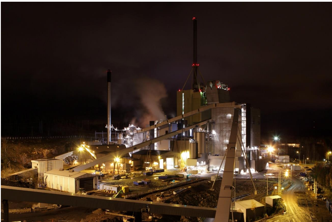
Figure 76 The Kymijärvi II plant at night. Conveyors to the gasifier building, the coal plant at its roof- located stack at the rear 397 .
